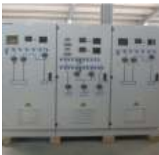
Low voltage DC and AC distribution panel (400/220/110kV). Transelectrica's Braşov station - Romania.
