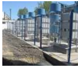
Medium voltage equalization capacitors coils and batteries with 6 adjustments steps used to compensate reactive energy (including harmonics filters). 52,4 MVar - Feral Tulcea - Romania.
