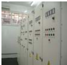
Low voltage DC and AC distribution panel (400/220/110kV). Transelectrica's Braşov station - Romania.
