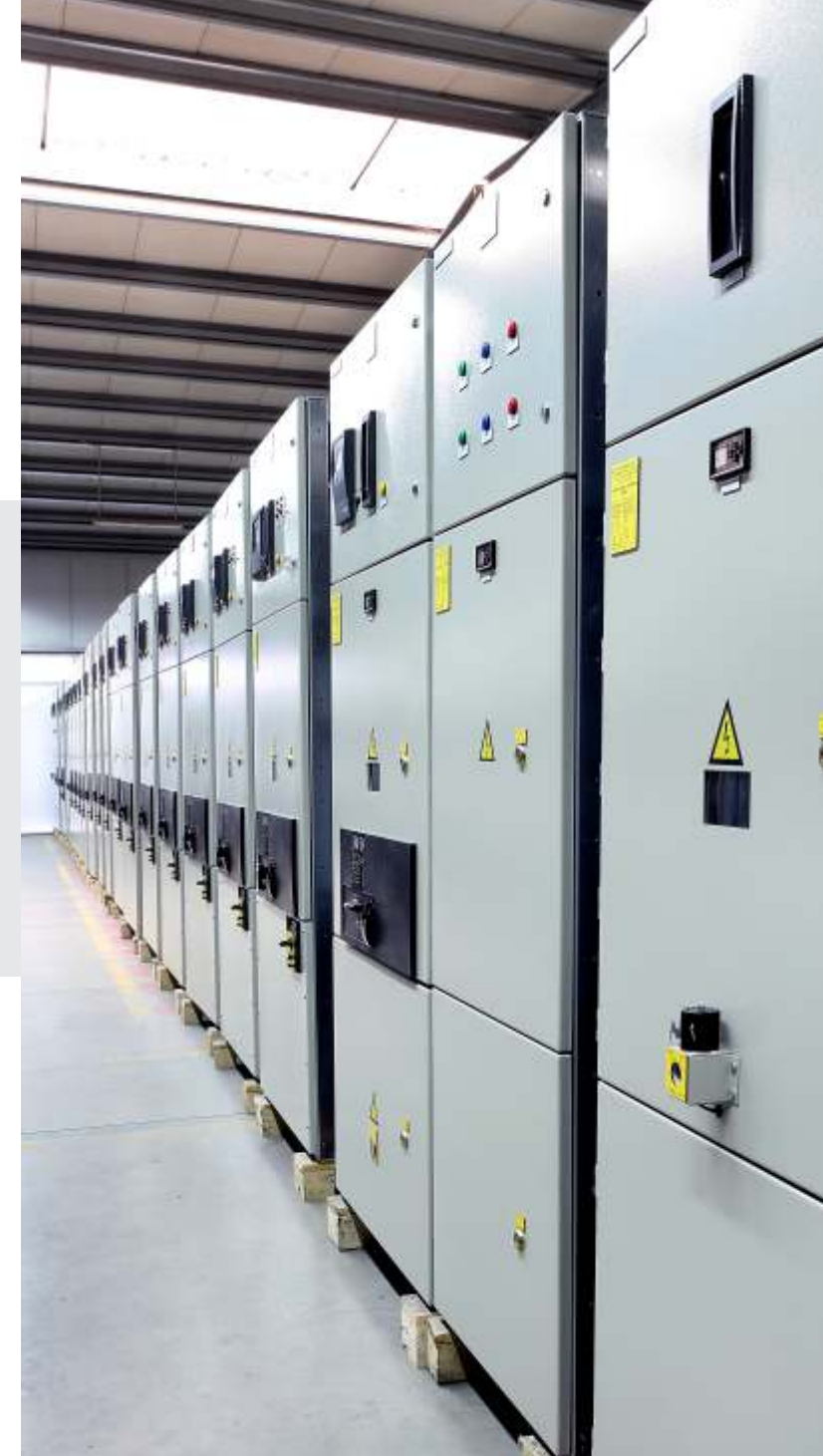
Medium voltage equalization capacitors coils and batteries with 6 adjustments steps used to compensate reactive energy (including harmonics filters). 52,4 MVar - Feral Tulcea - Romania.
