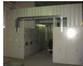
Medium voltage equalization capacitors coils and batteries with 6 adjustments steps used to compensate reactive energy (including harmonics filters). 52,4 MVar - Feral Tulcea - Romania.
